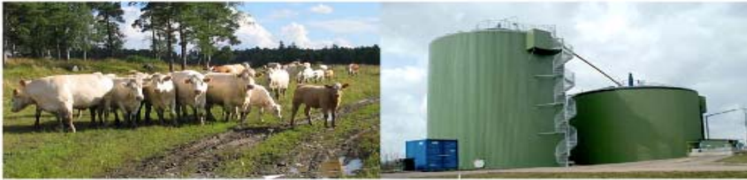
Figure 1. A biogas reactor can be started up using manure from cows or the contents of a digestion tank from an already operating biogas process. Photo Anna Schnürer
